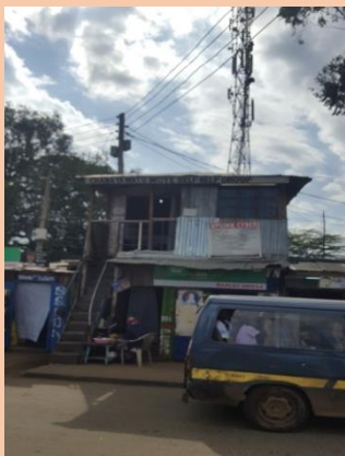
Before the demolition in 26 April 2018
