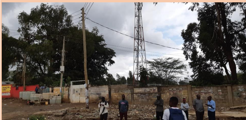
After the demolition in June 2018
